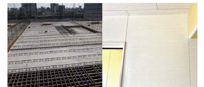
Precast concrete slab construction example
