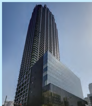
2009 The Kitahama ● 54-storied ultra-skyscraper condominium
