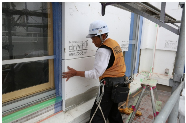
[外壁の工事風景]
