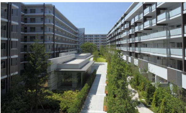
A pathway space in a rich green courtyard
