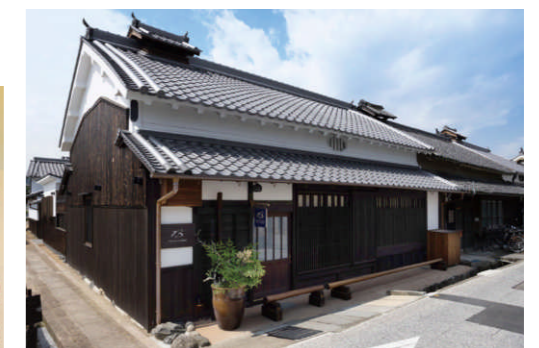
Accommodation facility in a restored old traditional house, “BRANCHERA VILLA ASUKA”
