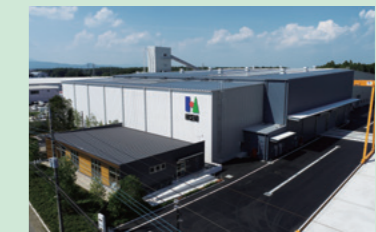
Precast concrete (PCa) plant
