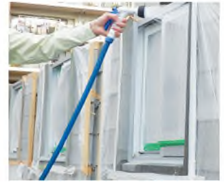
Window frame watertightness test
