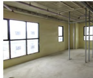
Spraying with thermal insulation material
