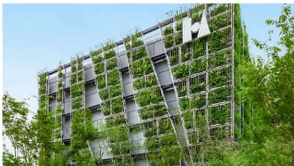
Green Wall of Multi-Purpose Laboratory building
