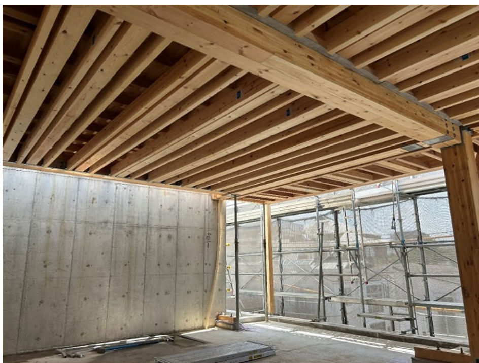
Construction site of Bransieta Meguro Chuocho, which uses wood (photograph taken in July 2024)
