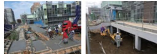
H-BA concrete construction scenery
