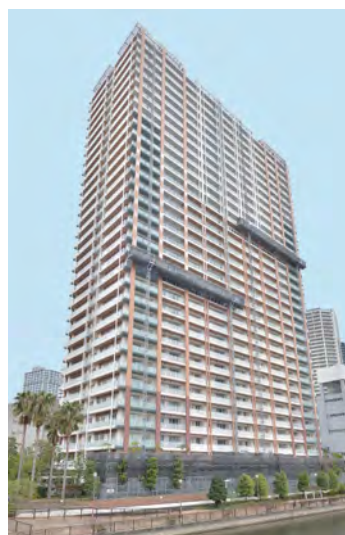
Large-scale repair: Lift-climber construction method
