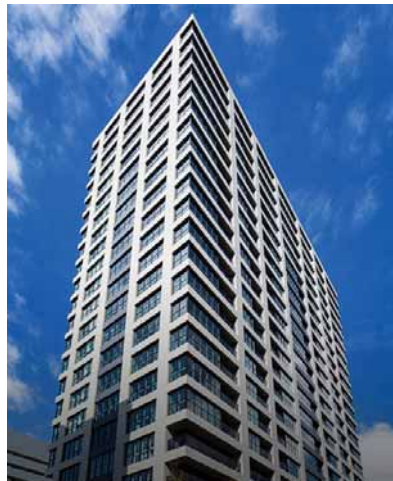
Laurel Tower Renai Hamamatsucho
