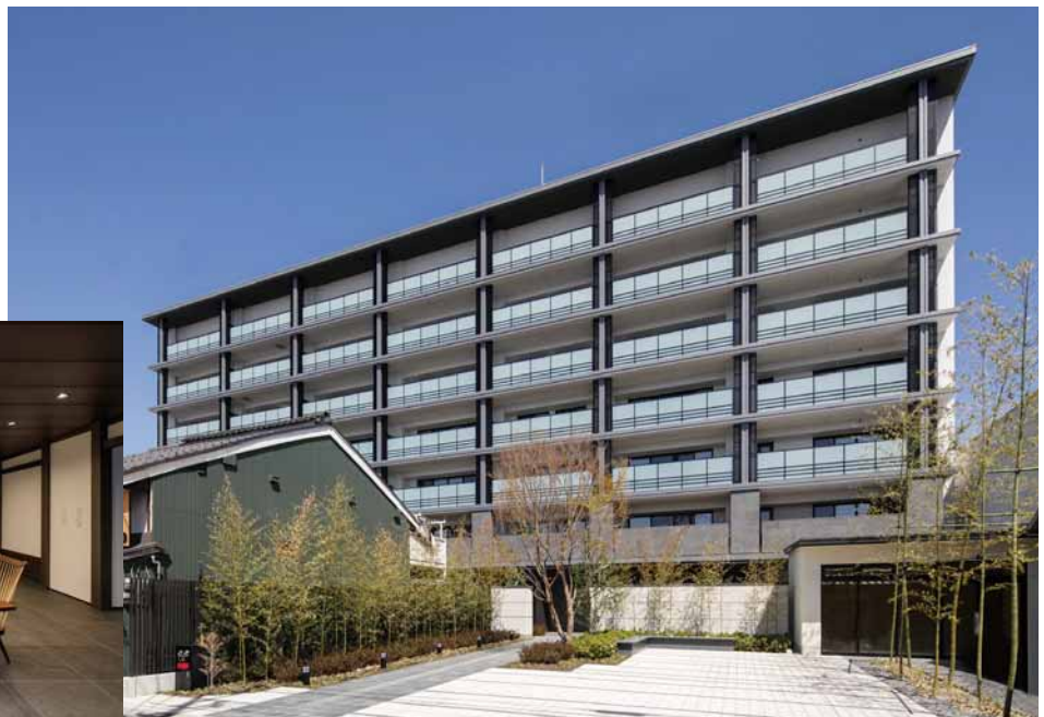
BRANCHERA Nagahama Motohamacho
