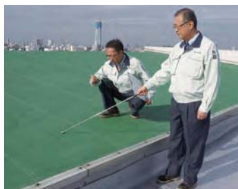
Building diagnosis by “Ju-yu-shi” (living-friendly engineers)
