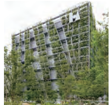
A multi-purpose test building with wall greenery effective for mitigating global warming and reducing CO 2 emissions
