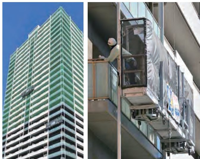
Large-scale repair: Lift-climber construction method
