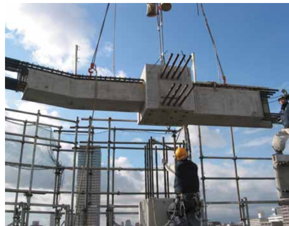
PCa beam construction
