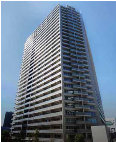
Prime Parks Shinagawa Seaside The Tower
