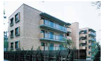
Palais Royal Midorigaoka Our first building replacement condominium
