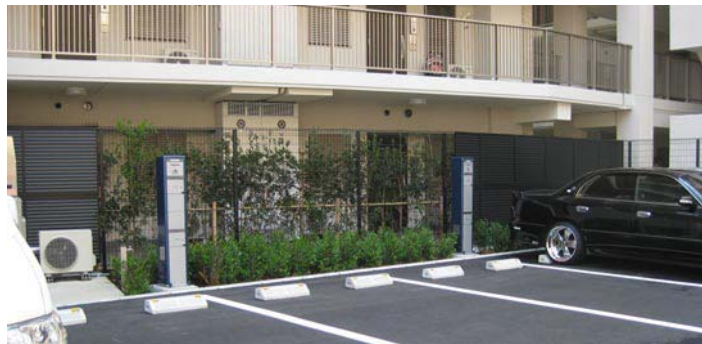
Installation of charging equipment dedicated to electric vehicles.
