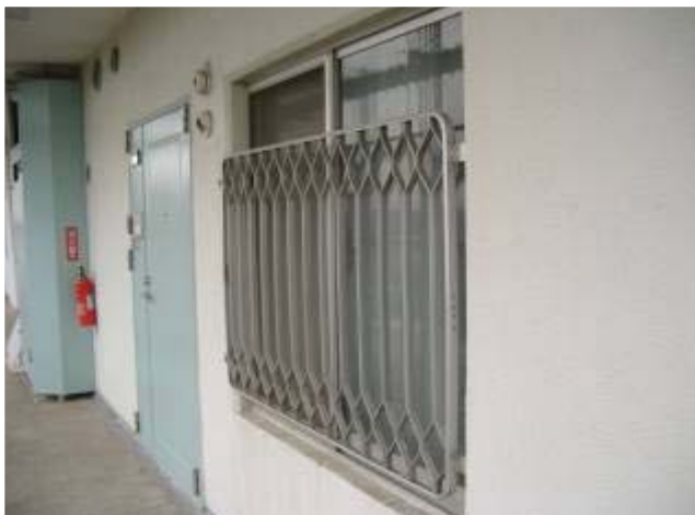
[リサッシ施工前]
