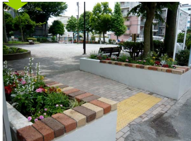
[改修後（西側入口）]
