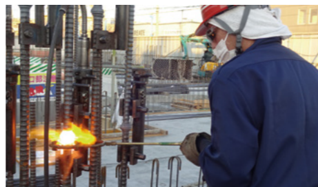
Adoption of natural gas pressure welding (Ecospeed Method)
