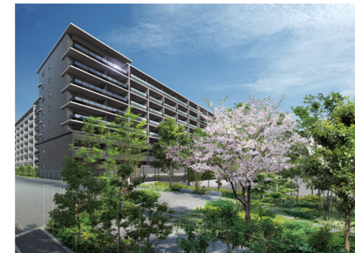
Exterior view of the southwestern side
