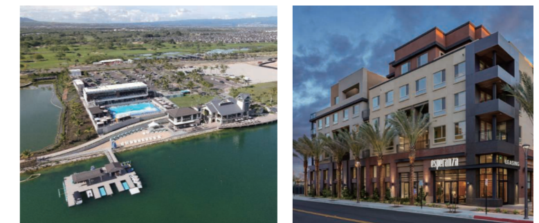
Complex facility Wai Kai
