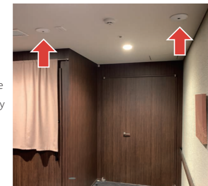
Cameras in front of the main bathroom count the comings and goings.
