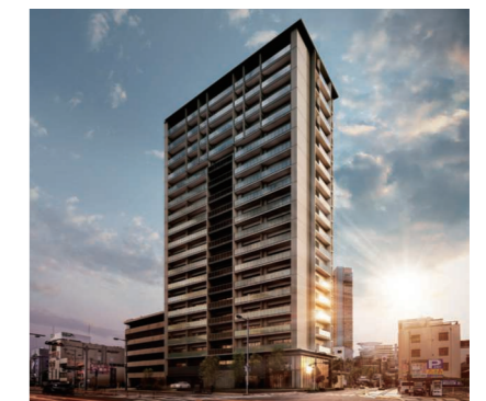
Branchera Takamatsu Nishinomaru Tower The Residence
