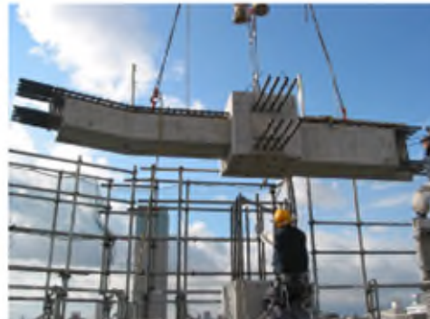
PCa beam construction
