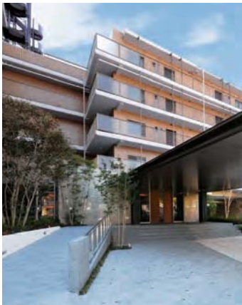
After (Enlargement of the slope)
