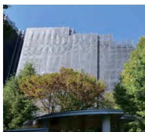
Large-scale repair: Under construction
