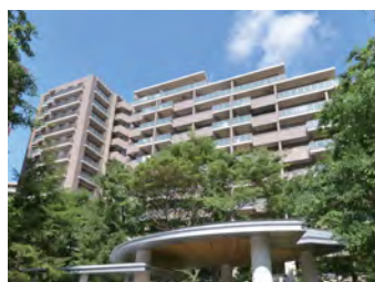
Large-scale repair: After construction
