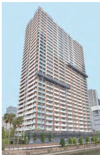
Large-scale repair: Lift-climber construction method
