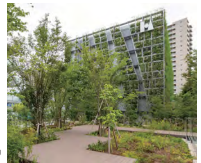
A multi-purpose test building with wall greenery effective for mitigating global warming and reducing CO 2 emissions
