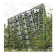
A multi-purpose test building with wall greenery effective for mitigating global warming and reducing CO<sub>2</sub> emissions
