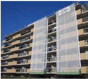
Modular type suspended scaffolding that secures anti-crime performance and livability
