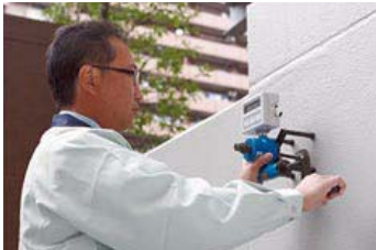
Building diagnosis by “Ju-yu-shi” (living-friendly engineers)
